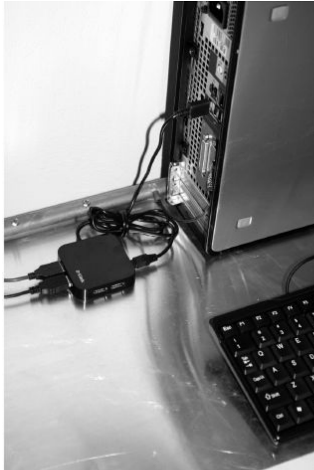
Figure 5.7 — Many inexpensive audio and computer accessories do not have metal enclosures and cannot be effectively connected to the RF ground plane or bonding bus. For this equipment, place the equipment and any attached cables directly on the ground plane. Note that DB-style connectors are often bonded to an enclosure. Use a multimeter to check for continuity between the connector's mounting screws and the power system ground conductor.
