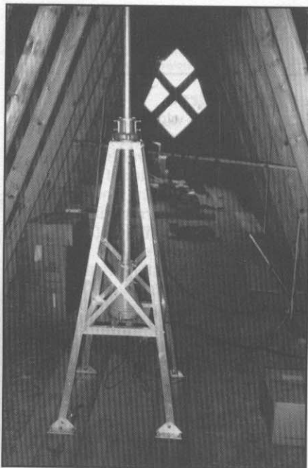
Fig 1—Four-legged roof-mount tower bolted to attic floor at K8KS. Two parallel, 6-foot lengths of 2×8-inch boards support the tower. These boards are, in turn, bolted to all the floor joists they contact. See text for details of the noise-reduction methods in use in this installation.
