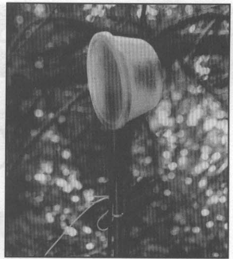
Fig 7—This is the complete weatherproof assembly for the coaxial cable connection at the antenna feed point.
