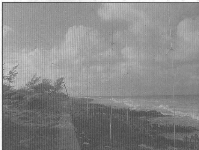
Fig 10 —Photo looking along the beachfront of the 1998 6Y2A operation from Jamaica. In the foreground is the two-by-two vertical half-wave array for 15 meters into Europe. The 10-meter two-by-two array is behind this, and the two-element horizontal 20-meter Yagi at 30 feet shows up in the background.
