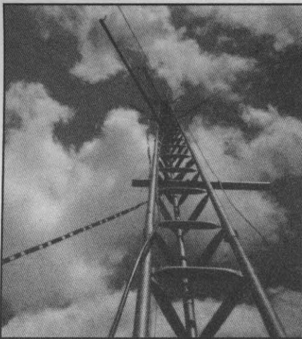
Fig 2—Photo looking up the 160-meter tower.
