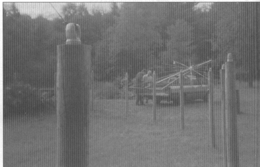
Fig 10 —Photo showing some of the fence posts used to hold individual cone wires to keep them off the ground and out of harm's way. The truck in the background is carting away the A-frame discone for installation at KA8UNO's QTH.
