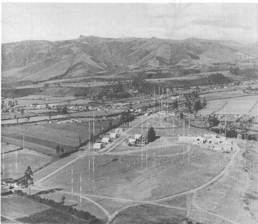
Fig 1—Radio heaven or radio hell? The antenna system of HCJB, near Quito, Ecuador, was located literally in the author's backyard! His house is at the center of the photo, the top building in the row of four.
