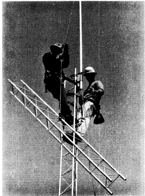
Fig. 14-9 — The assembly of tower sections is made simple when a gin pole is used to lift each one into position. Note that the safety belts of both climbers are fastened below the pole thereby preventing the strap from slipping over the top section. (Photo by K1THQ)
