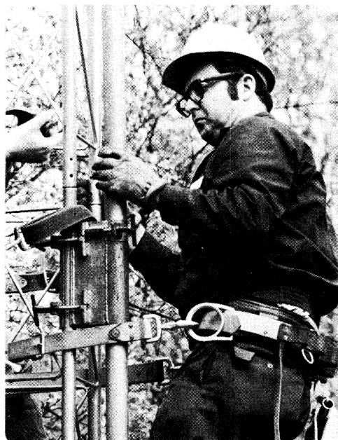
Fig. 14-13 — A good-quality safety belt is a requirement for working on a tower. The belt should contain large steel loops for the strap snap. Leather loops at the rear of the belt are handy for holding tools. (Photo by K1THQ)
